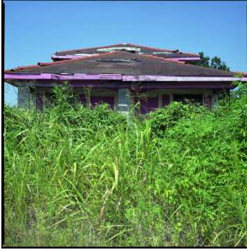
Katrina Damage House, 2010
